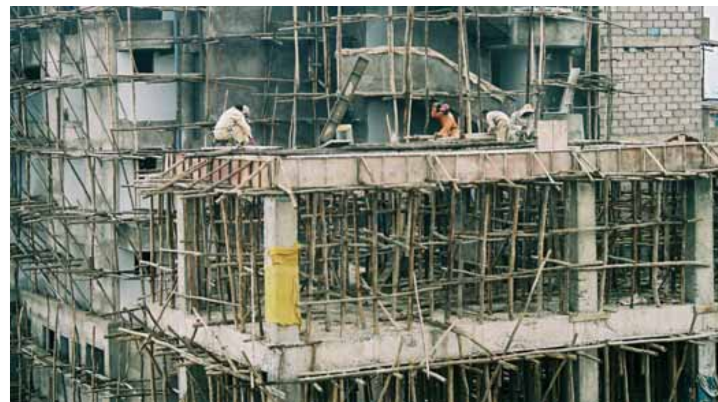
Construction workers on an Addis Ababa building site. © François Misser
