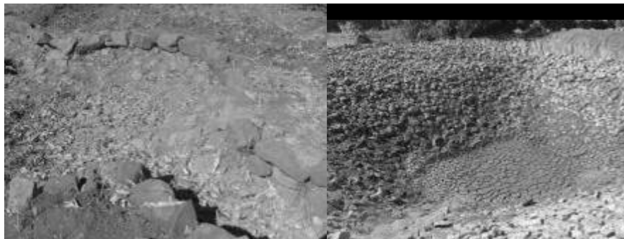
Picture 11. Silt trap structure and silt deposit in pond
