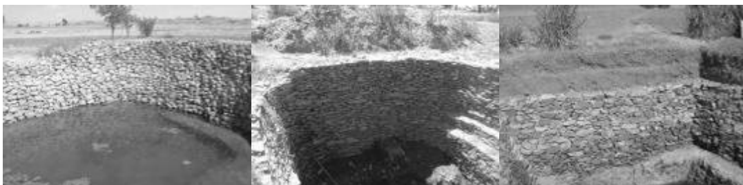
Picture 3. Structural view of hand dug shallow wells
