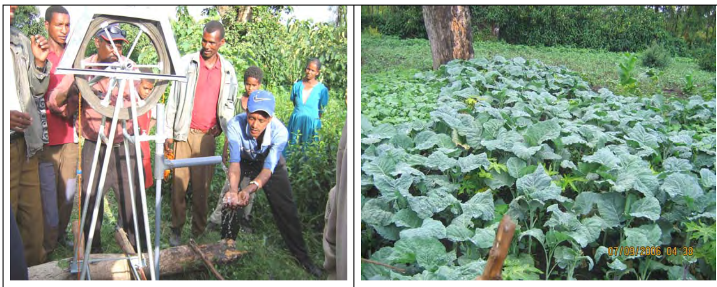
Rope pump installation and vegetable gardening in Yimer Wacho kebele, (Meskan)
