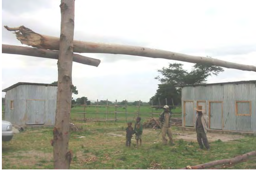
Generator house, office and storerooms of Simbita bore hole water supply scheme
