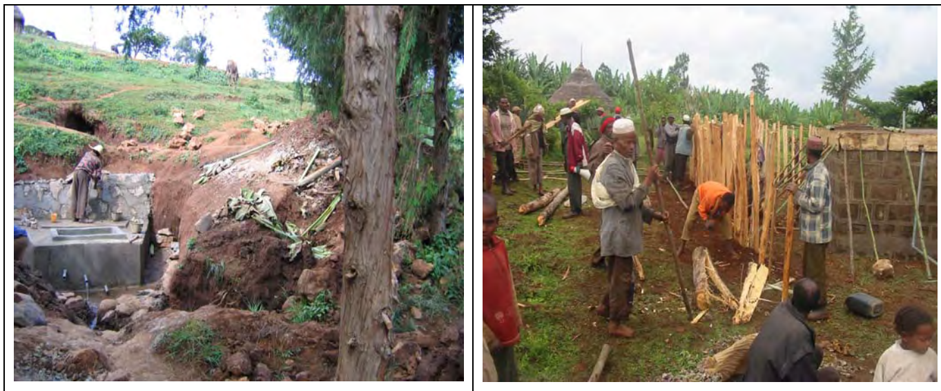
Anshebesso spring development (Siltie)
