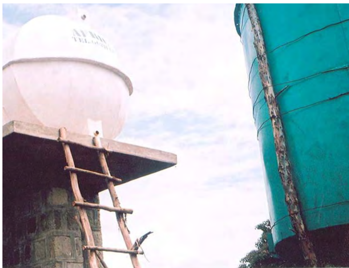
Water reservoir (white fiber glass), and de-fluoridation tank (blue sheet metal) for Sinbita water supply scheme
