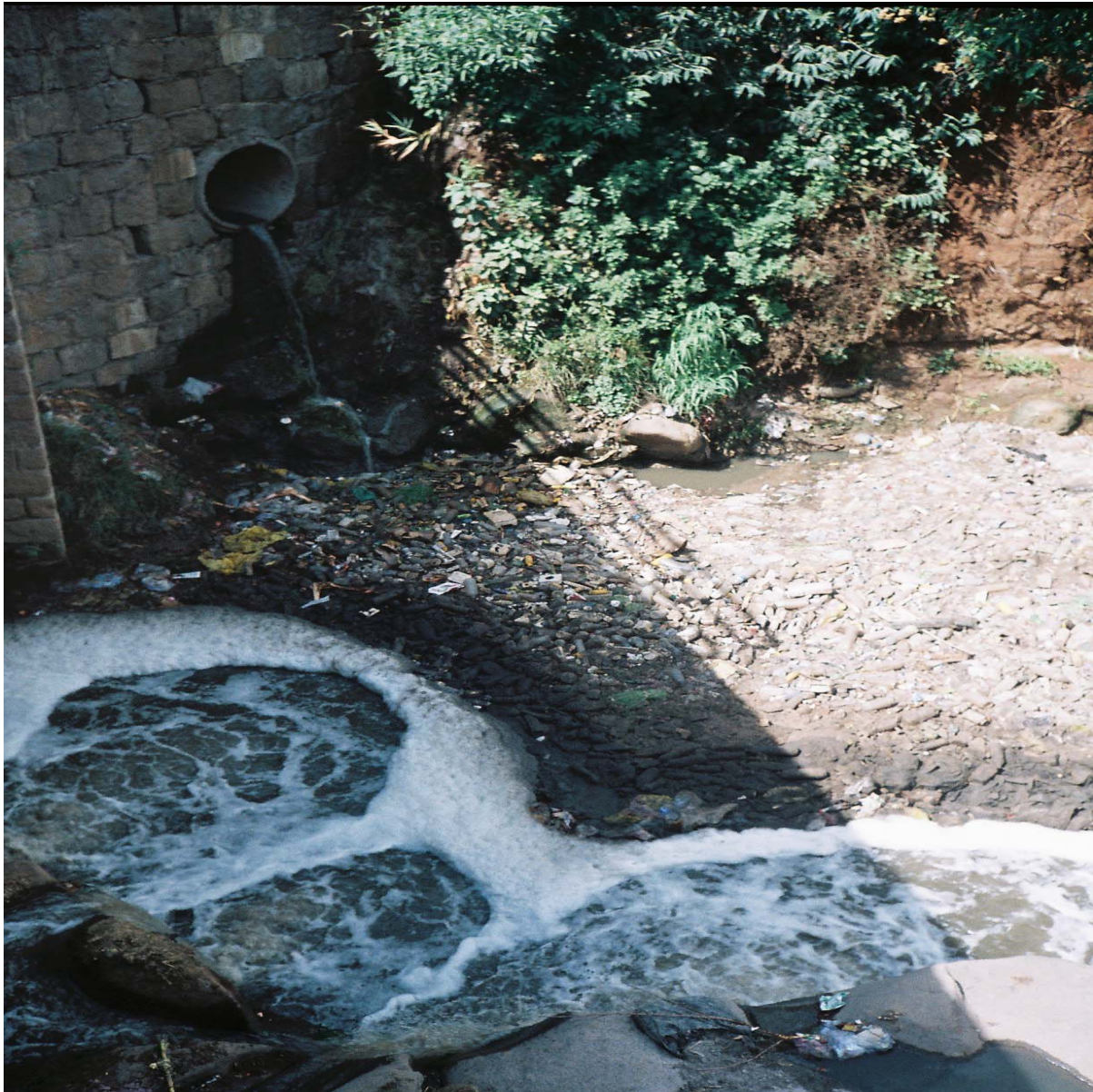
Fig.10 Storm Drain Feeding Tributary Shankla at a bridge near Ethiomarble.
